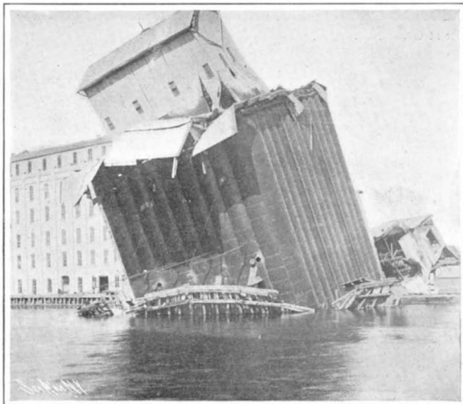
A GRAIN ELEVATOR WHICH GLIDED INTO A RIVER AFTER ITS FOUNDATION FAILED.
