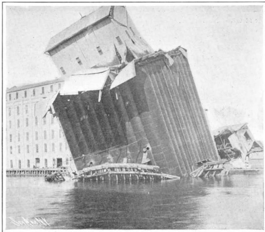
A GRAIN ELEVATOR WHICH GLIDED INTO A RIVER AFTER ITS FOUNDATION FAILED.
