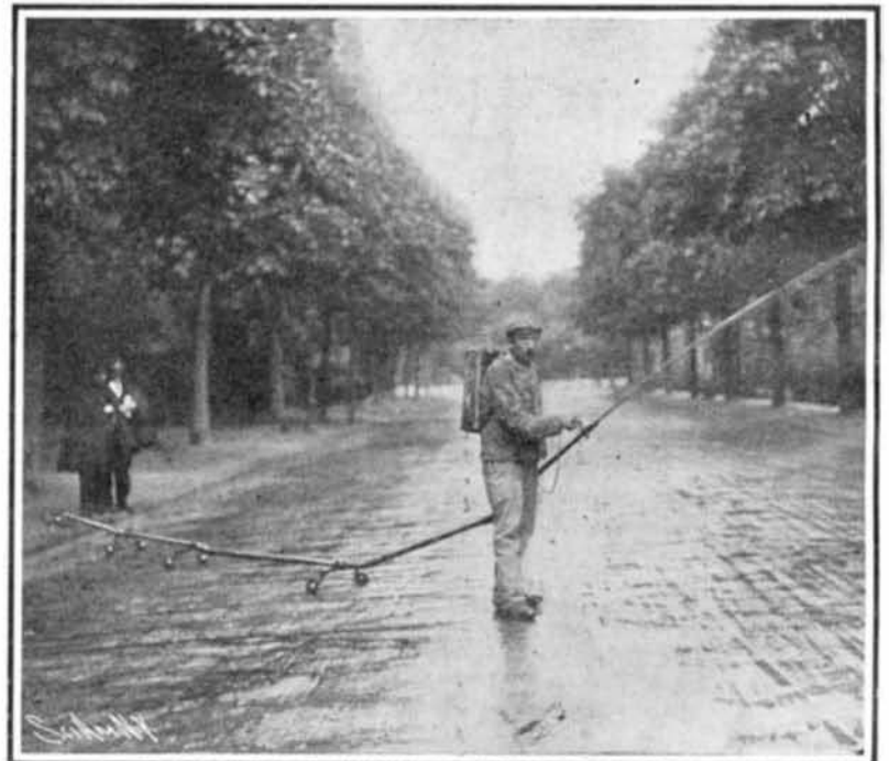
One Way of Applying Tar or Oil Consists in Piping the Water from the Mains Through a Hose. Oil or Tar is Fed to a Special Nozzle and Mixed with the Water.
