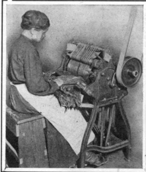
Fig. 5.—Stripping by Machinery. Operator Withdrawing Stripped and Booked Leaves.
