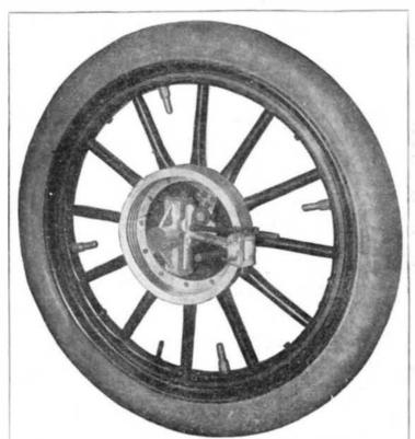
ALL experienced Automobilists are aware of the dangers and inconvenience of stopping and starting core of stopping and starting cars on an up grade, with the ordinary brakes now in use. The injury to machinery caused by throwing the clutch in too soon, in starting, and the danger of running backwards down hill, should the brakes be released too soon, makes the Hayden Automatic Back Stop an absolute necessity on every up-to-date car.
