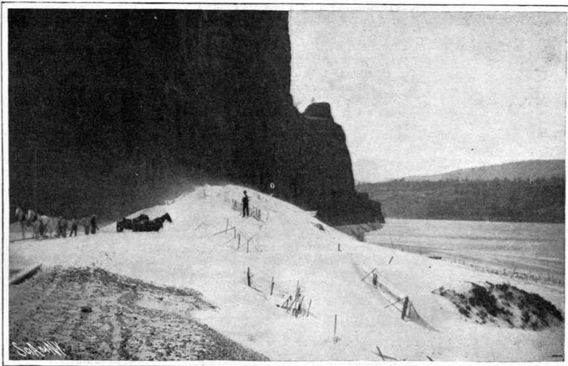
Railroad Men Fighting the Sand Sea in Oregon. The Track Can Be Seen to the Left Partly Buried.
