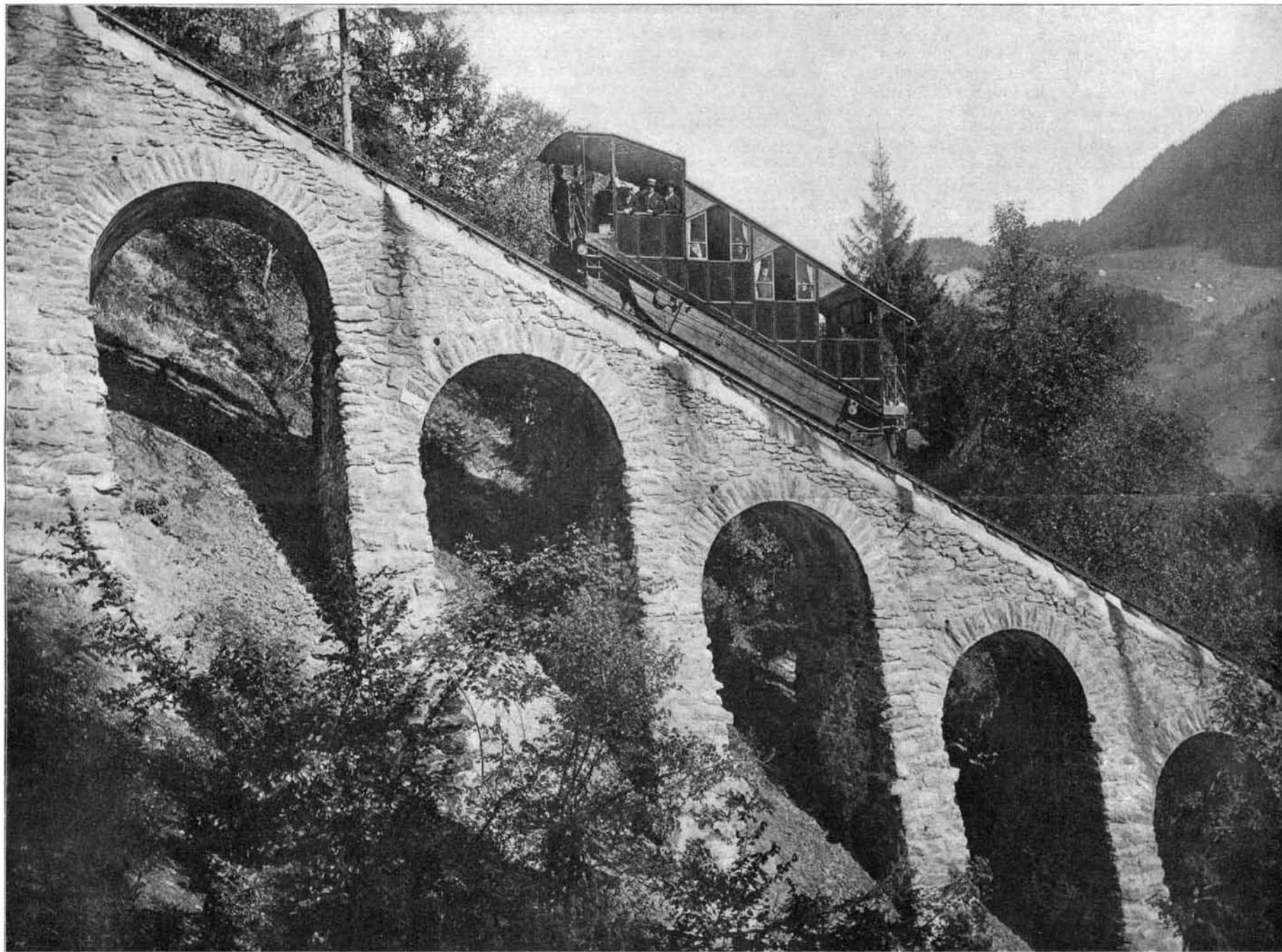
CAR CROSSING A STEEP VIADUCT ON THE LAUTERBRUNNEN-GRÜTSCH ALP GRAVITY CABLE RAILWAY.
