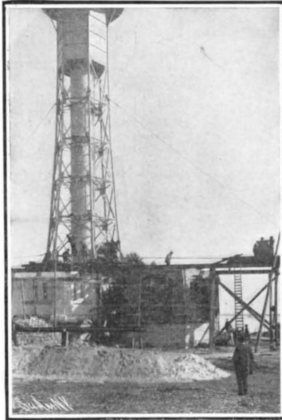
Lighthouse During Removal.
