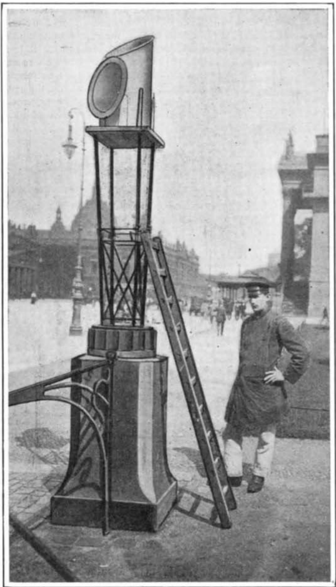
The Dust Collector Set up in a Prominent Square in Berlin.
