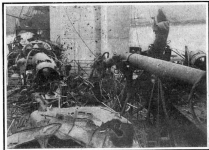
Wreckage on the Bridge Deck of the "Orel."
