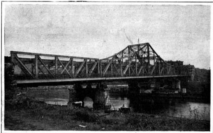
The New Drawbridge Span Located in Position.
