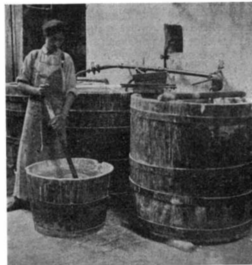
Fig. 2.—Mixing Colors with Stearine.
