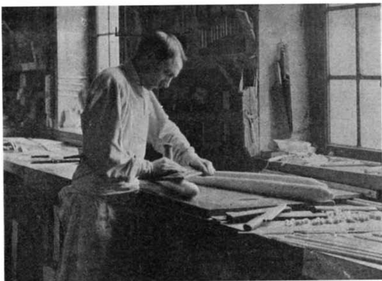
Fig. 5.—Rolling Wax Candles.
