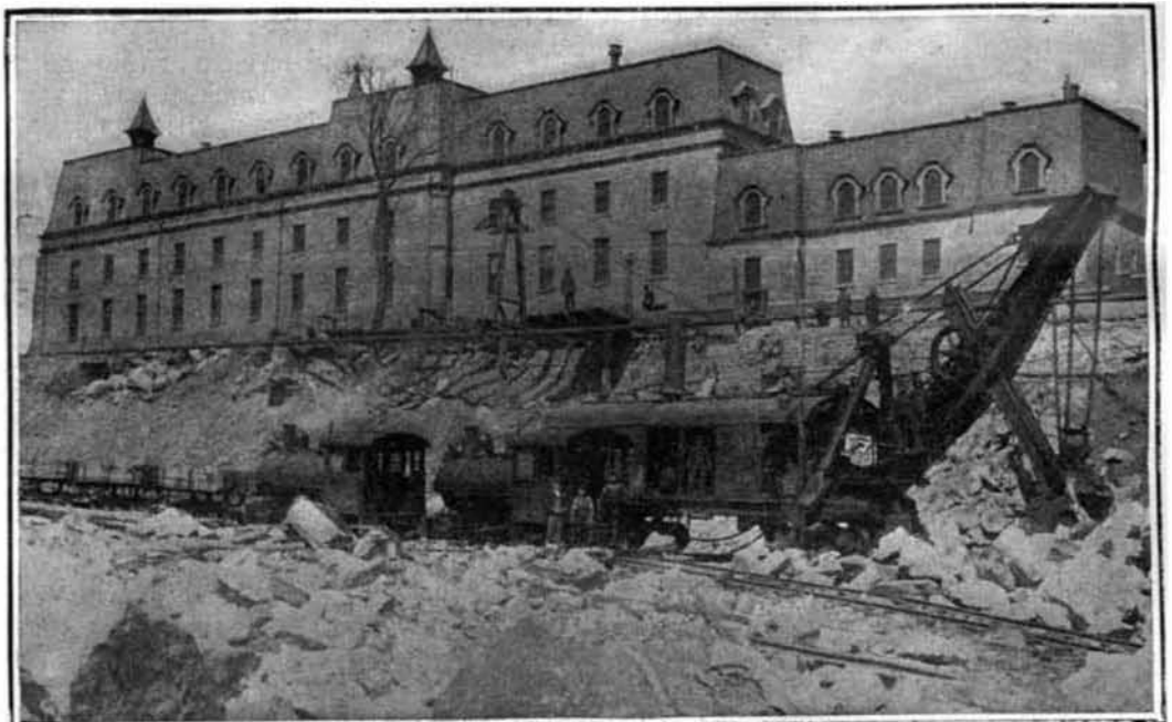
Seventy-Ton Steam Shovel Working on Northerly Side of Excavation at 33d Street.
