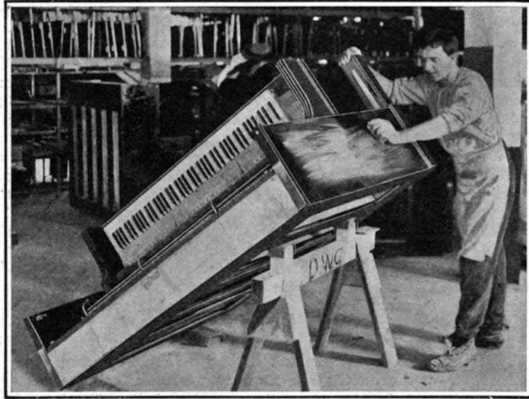
Polishing the Case. Rubbing Down with Powdered Pumice Stone.
