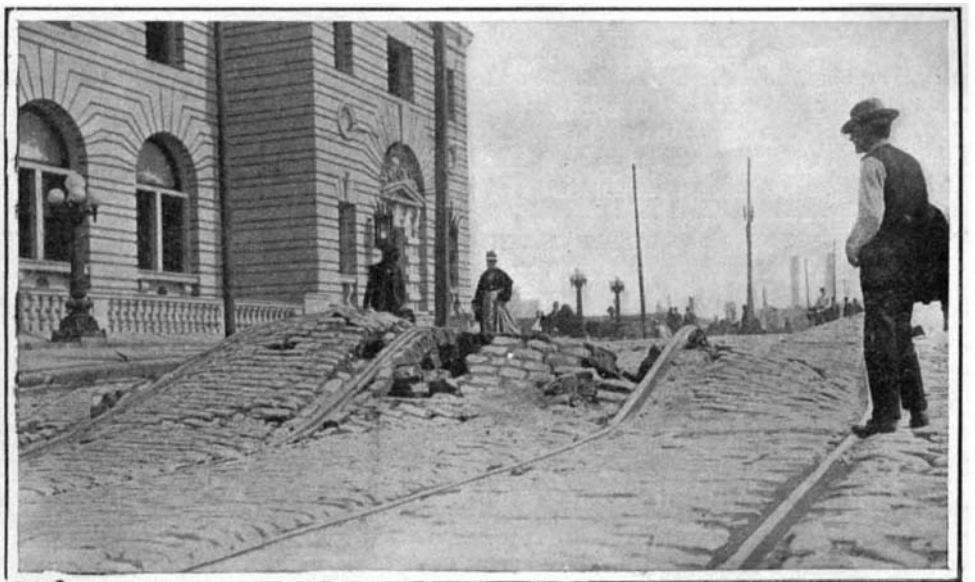
Street and Railroad Track Elevated by the Earthquake at the Post Office.
