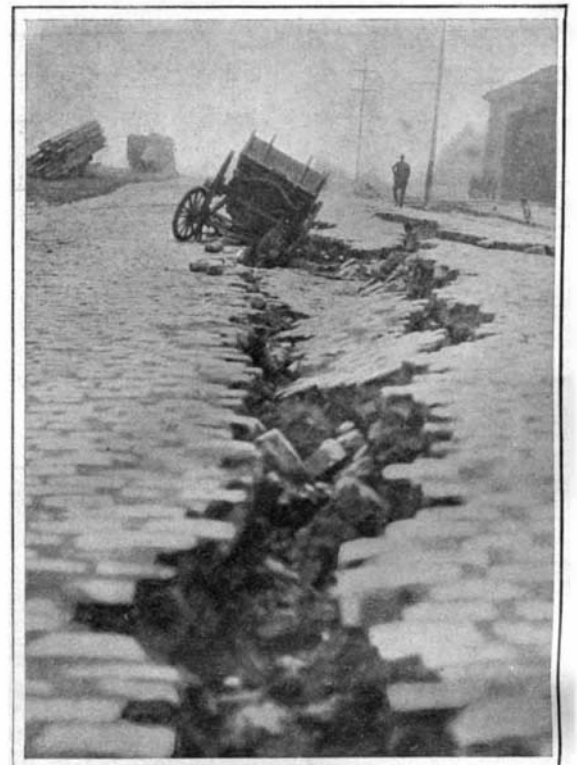
Fissure Produced by the Earthquake in a San Francisco Street.
