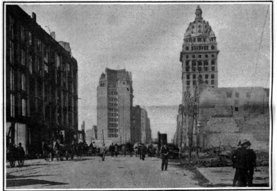
View Showing How Well Steel-and-Masonry Buildings Stood the Test of Earthquake and Fire.
