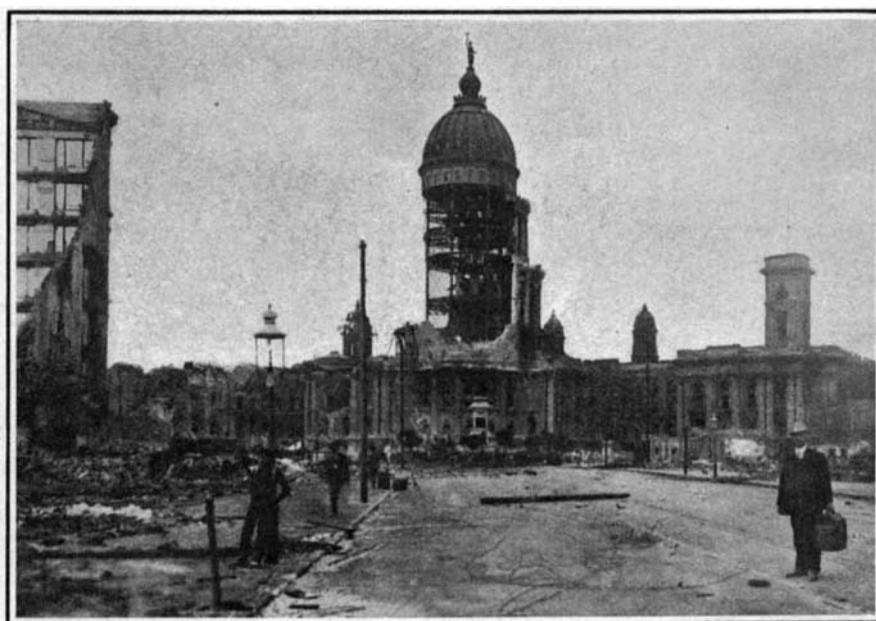
Effect of Earthquake on the City Hall, Showing Steel Frame and Dome Intact; But Masonry Thrown Down.
