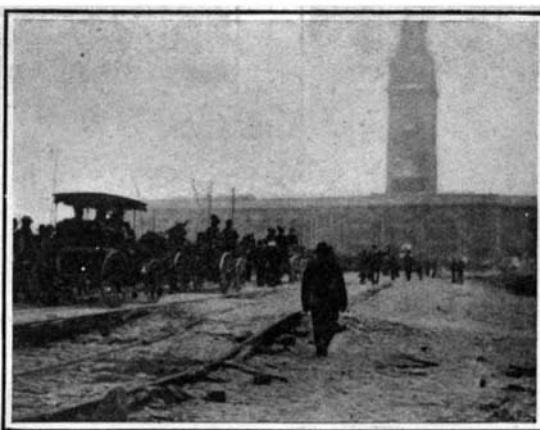
Crevice and Subsidence of Car Track.
