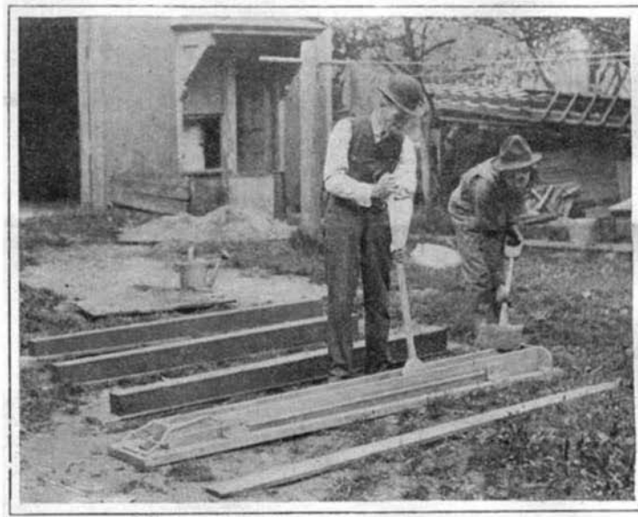
Fig. 8.—Making Concrete Fence Posts.
