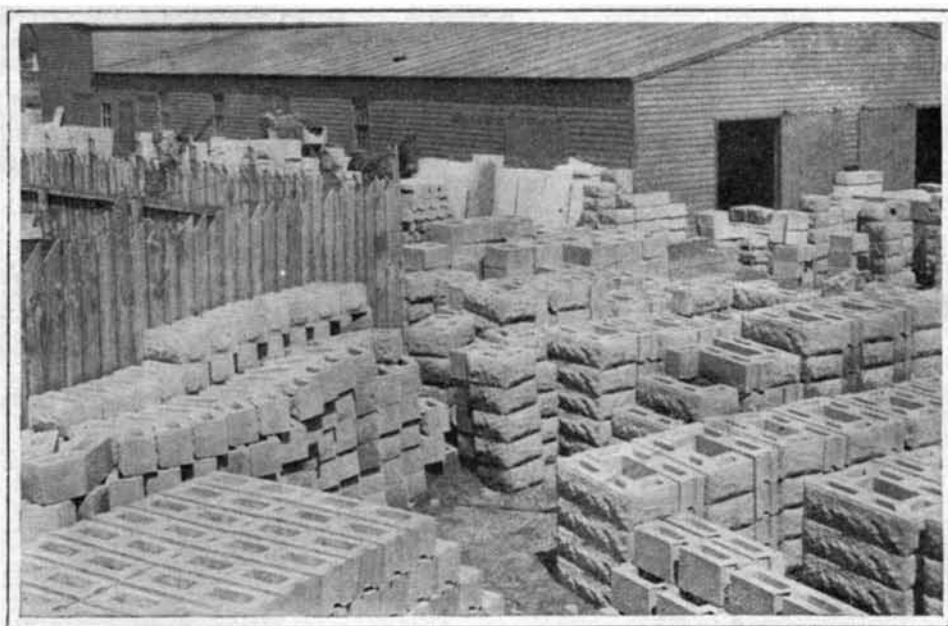
Fig. 5.—A Yard of Finished Concrete Blocks.
