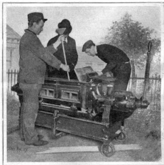
Fig. 2.—Tamping Concrete in Hayden Machine.
