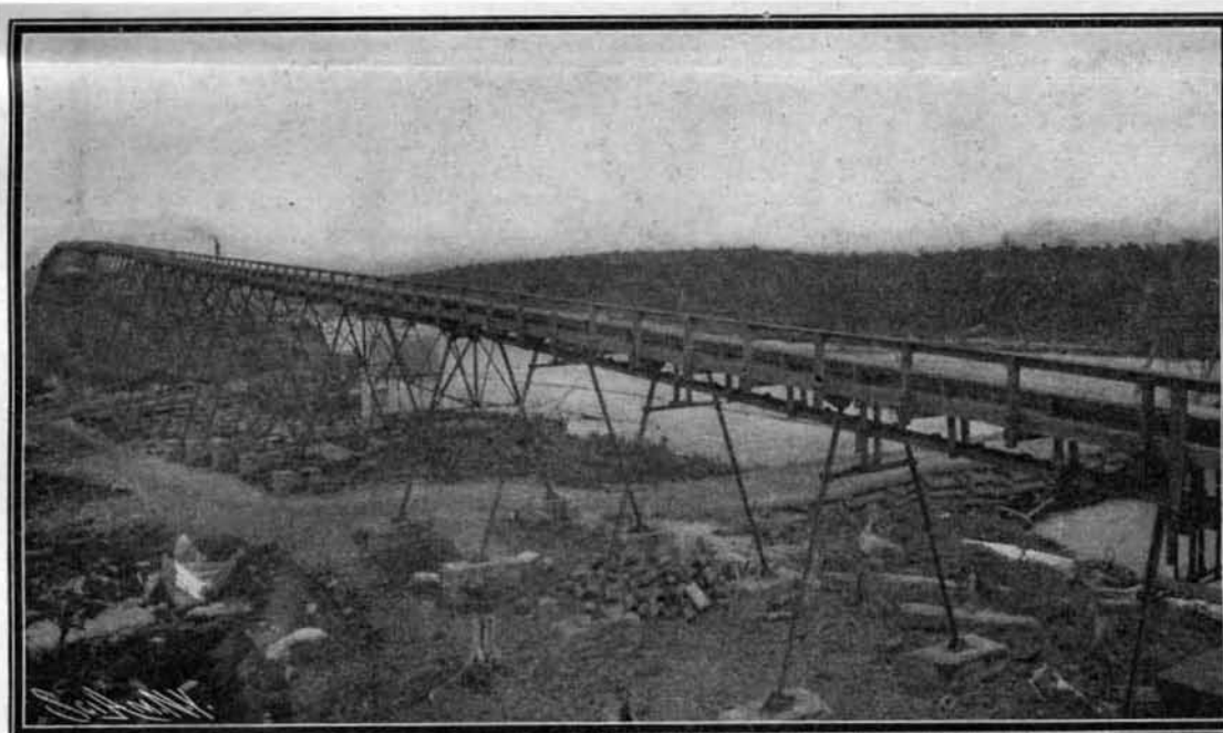
Type of Heavy Conveyer for Hauling Logs to Sawmill.
