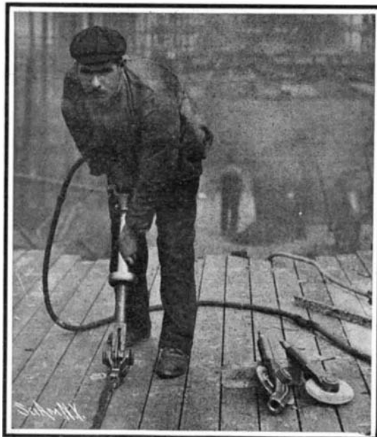
PNEUMATIC DECK-CALKING TOOL IN OPERATION, SHOWING SEAM OPENER AND CALKING IRON WITH PNEUMATIC HAMMER.
