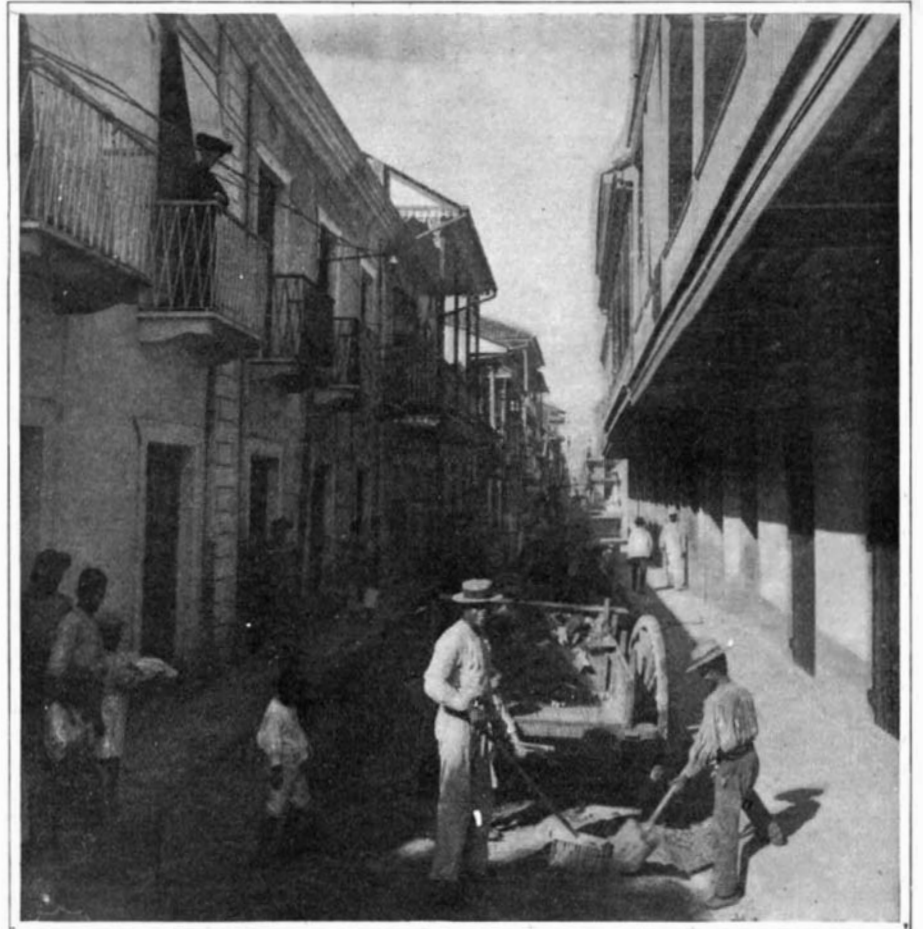
Street Cleaning Department at Work on One of the Streets of Panama. This Street Has Been Graded and Covered with Top Dressing of Gravel.
