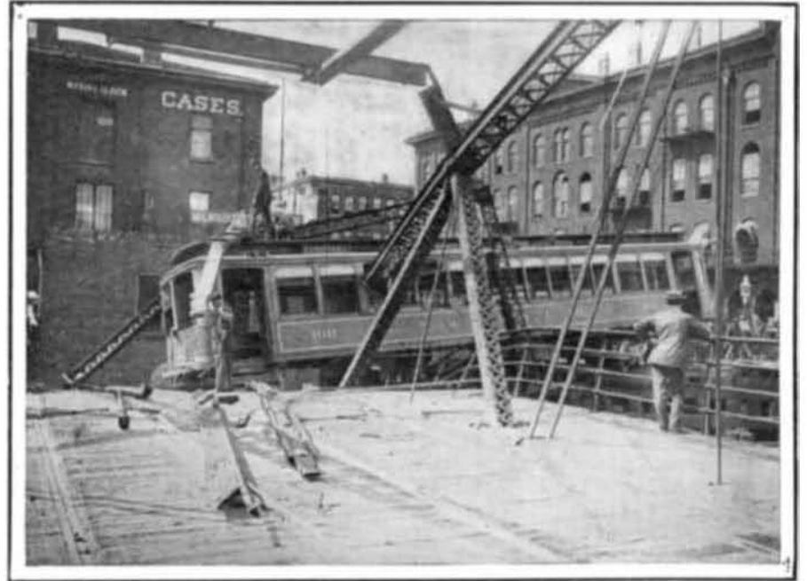
After the Collision; the Car is Resting Partly on the Bridge and Partly on the Street.
