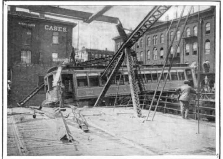
After the Collision; the Car is Resting Partly on the Bridge and Partly on the Street.
