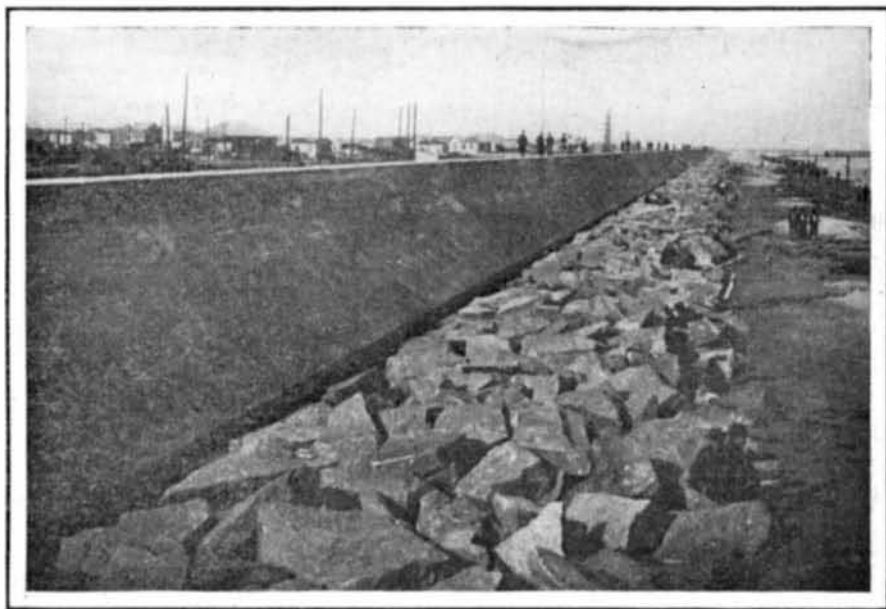
BUILT OF GRANITE AND CEMENT, THE GALVESTON SEA WALL IS 4½ MILES LONG AND WEIGHS 40,000 POUNDS TO THE FOOT.
