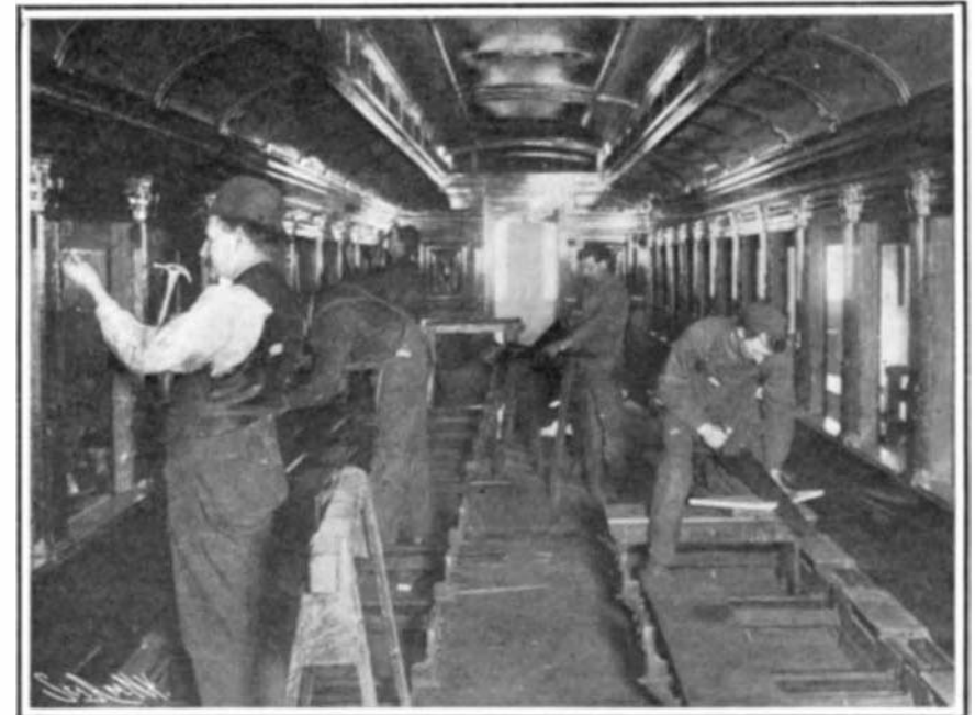
Nailing on the Hardwood Finishing.
