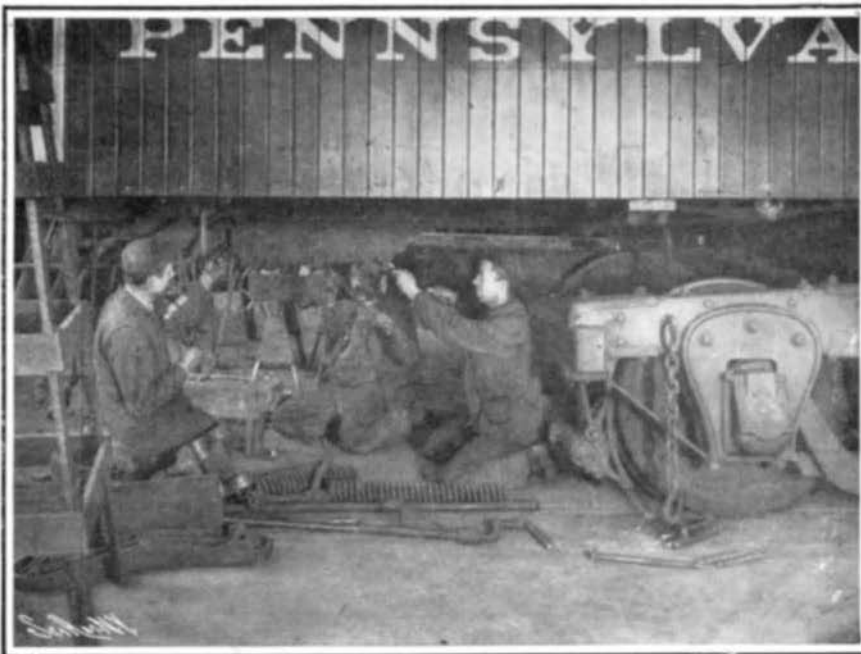
Fitting a Truck to a Completed Car Body.
