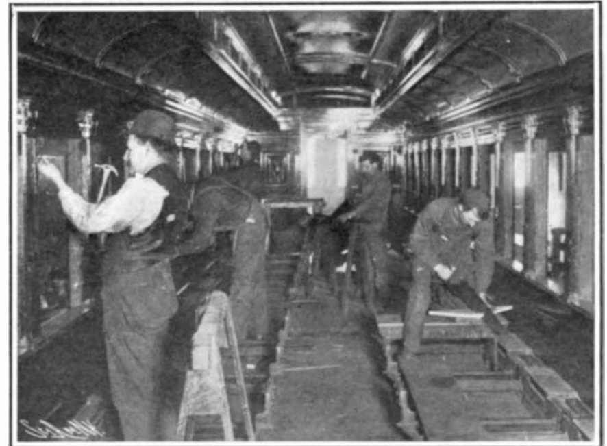
Nailing on the Hardwood Finishing.
