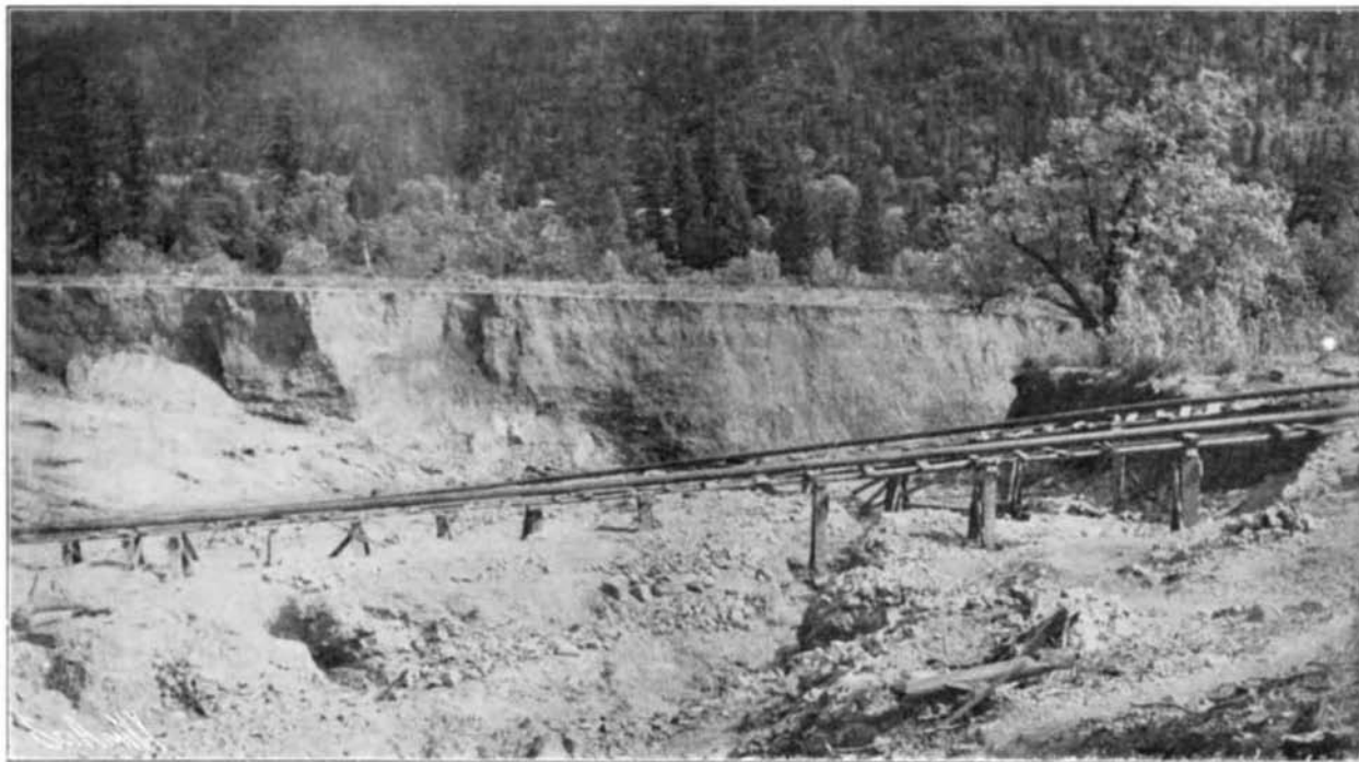
The Pipe Line from the Pumps to the "Giants." HYDRAULIC MINING WITH CENTRIFUGAL PUMPS.
