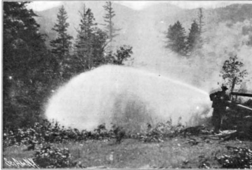
"Giant" in Operation, Throwing Stream 250 Feet.
