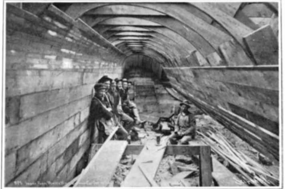
Interior of Wooden Form for Concrete Wing-Dam.
