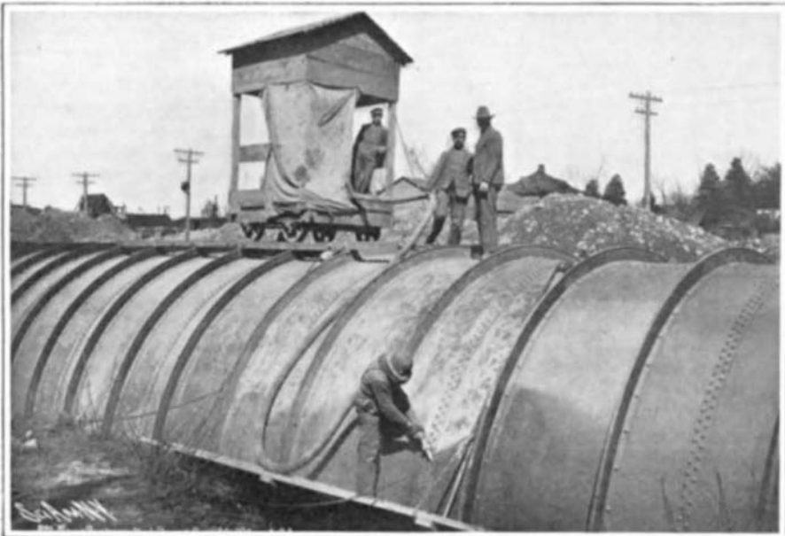
Sand-Blasting One of the 18-foot Steel Conduits.
