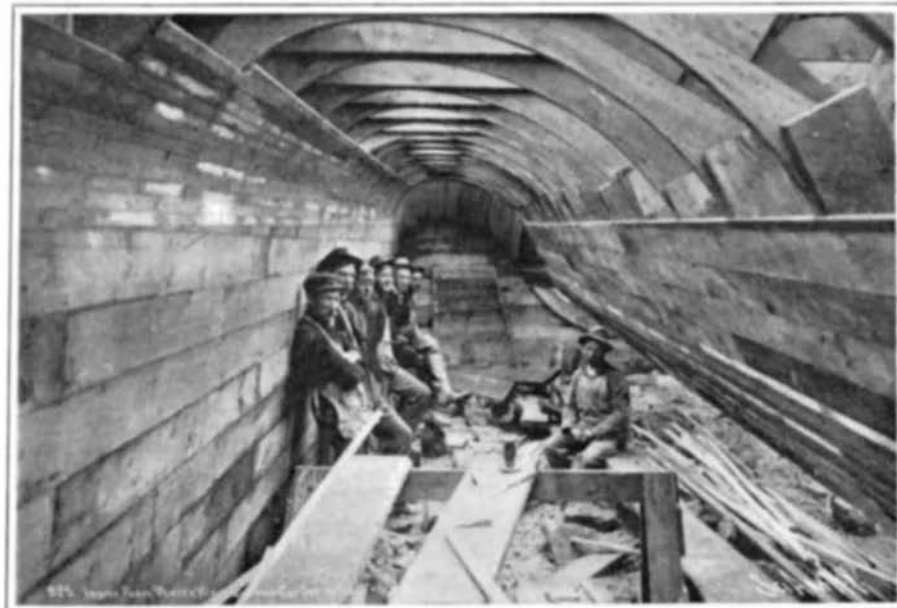
Interior of Wooden Form for Concrete Wing-Dam.
