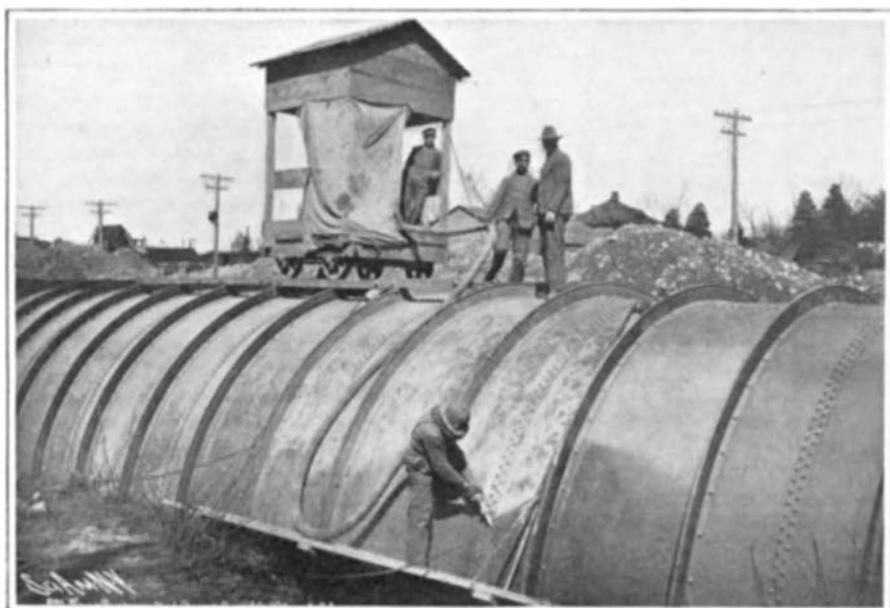
Sand-Blasting One of the 18-foot Steel Conduits.
