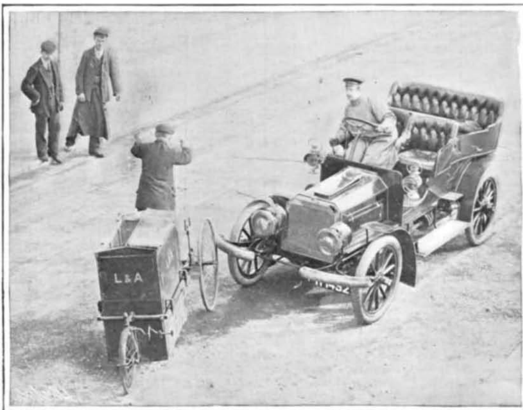
Car Equipped with Buffer Striking a Delivery Tricycle.
