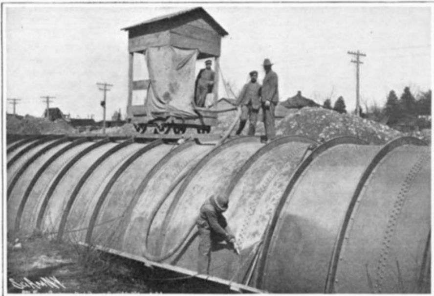
Sand-Blasting One of the 18-foot Steel Conduits.
