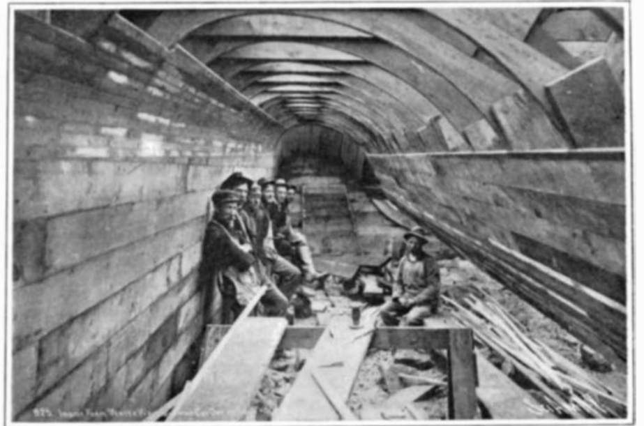
Interior of Wooden Form for Concrete Wing-Dam.
