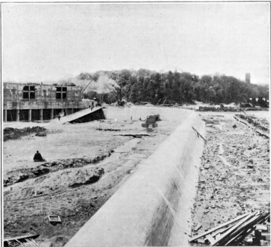
Concrete Wing-Dam for Gathering the River Water into the Forebay.
