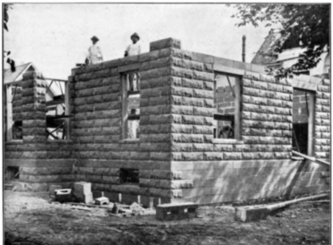
LAYING HOLLOW CONCRETE BUILDING BLOCKS.
