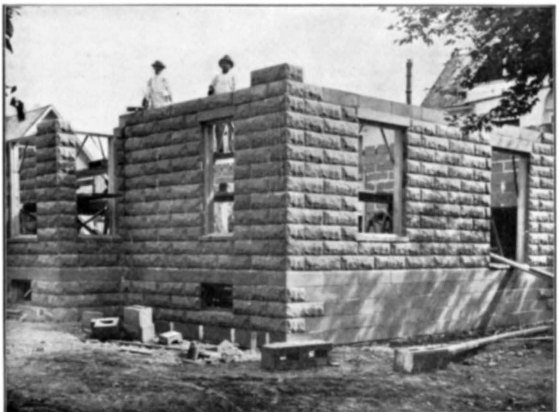
LAYING HOLLOW CONCRETE BUILDING BLOCKS.
