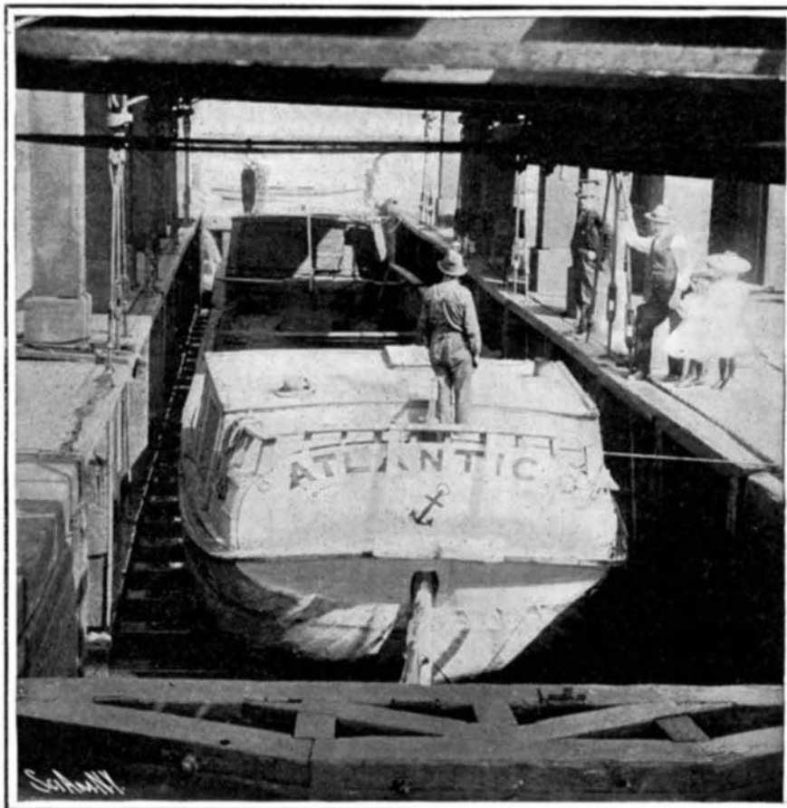
WEIGHING A CANAL-BOAT IN THE CLEVELAND LOCK.
