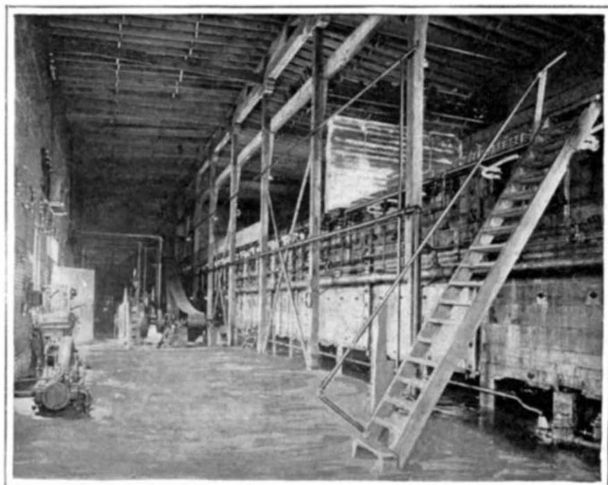
Interior of the Plant, Showing Tank to the Right with Cake of Ice Being Lifted by the Electric Crane.
