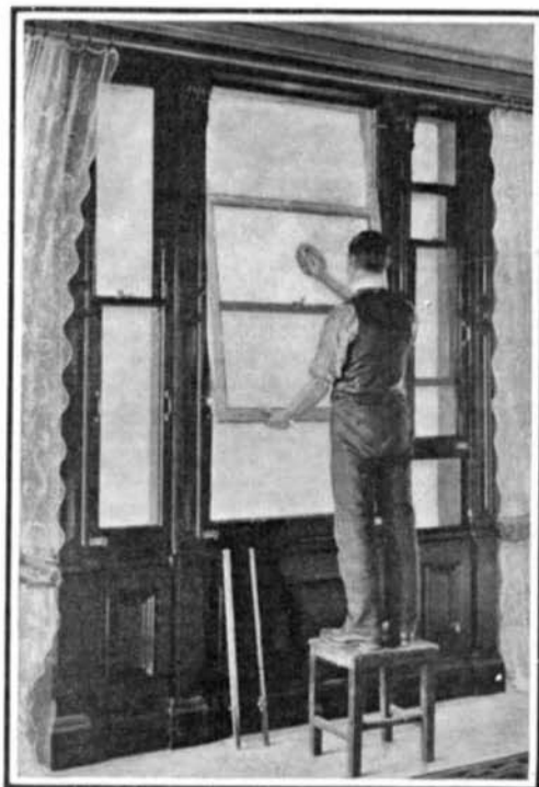
Top Sash Swung in for Cleaning.
