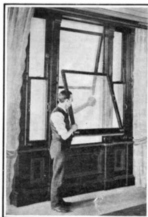
Cleaning the Lower Sash.
