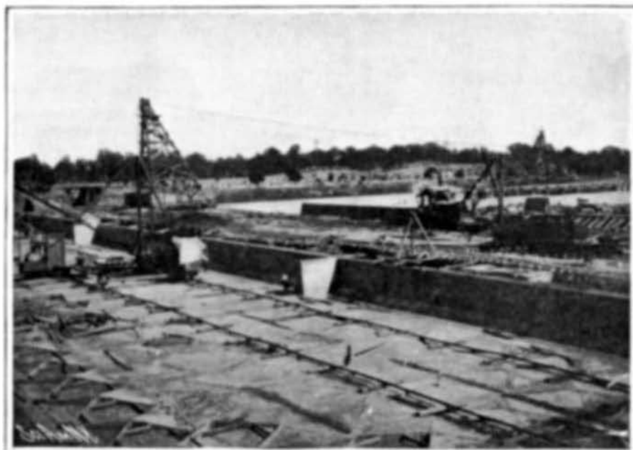
Construction Work of Filtration Plant.
