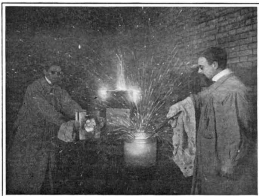
When the Furnace Has Done Its Work the Crucible, White Hot, is Plunged into Melted Lead or Cold Water. The Sudden Contraction and Consequent Pressure Produce the Diamond.
