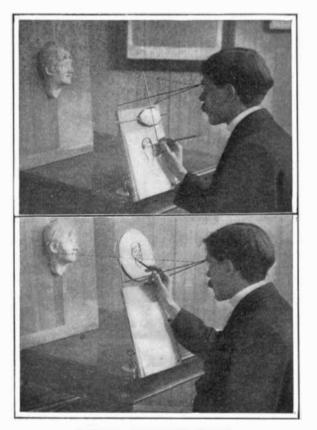
the other in which a pantographic attachment is used. The latter is shown in the upper illustration. The device consists of a drawing board which may be fastened to the edge of a table by means of a clamp. Attached to the drawing board is a wire frame which, at its outer end, is bent into a ring to which the eye of the artist is applied. The pantographic device comprises a horizontal fixed rod which carries a metal
