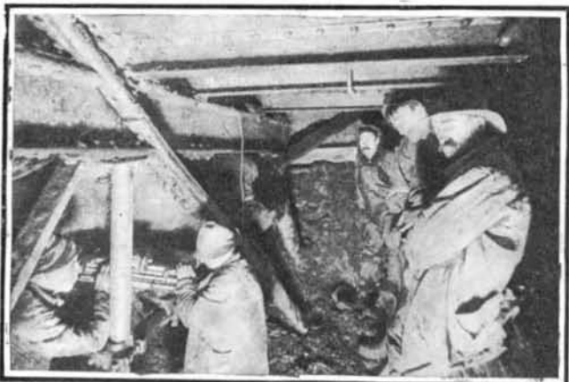
View Beneath the Apron Used in Front of Shield in Removing Rock Obstructions.
