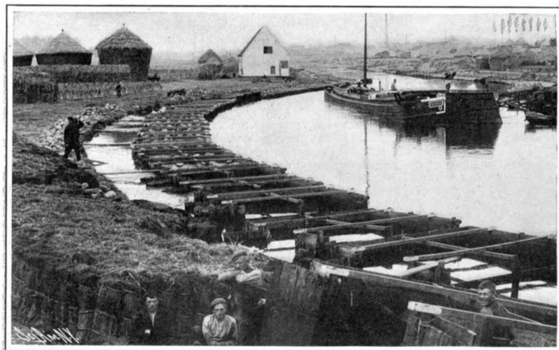
Crates of Flax Weighted and Sunk in the River Lys.
