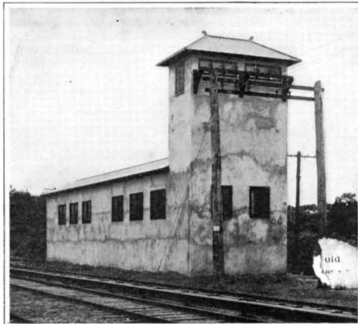
Steel and Concrete House for Housing Two Portable Sub-Stations.
