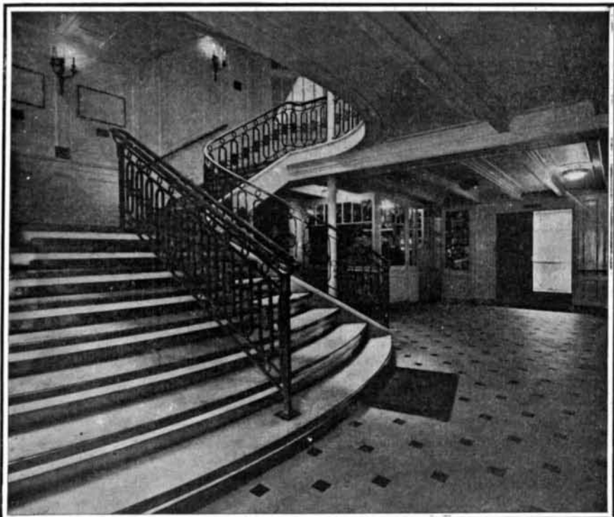
Main Stairway, Showing Florist's Store in the Far Corner.
