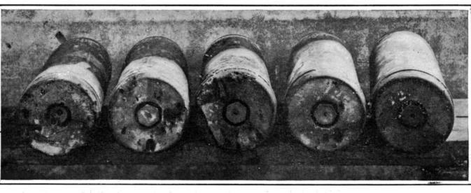
Five Shells, Carrying Pressure Gages in the Base, Showing Scoring by Fragments of the Shell.
