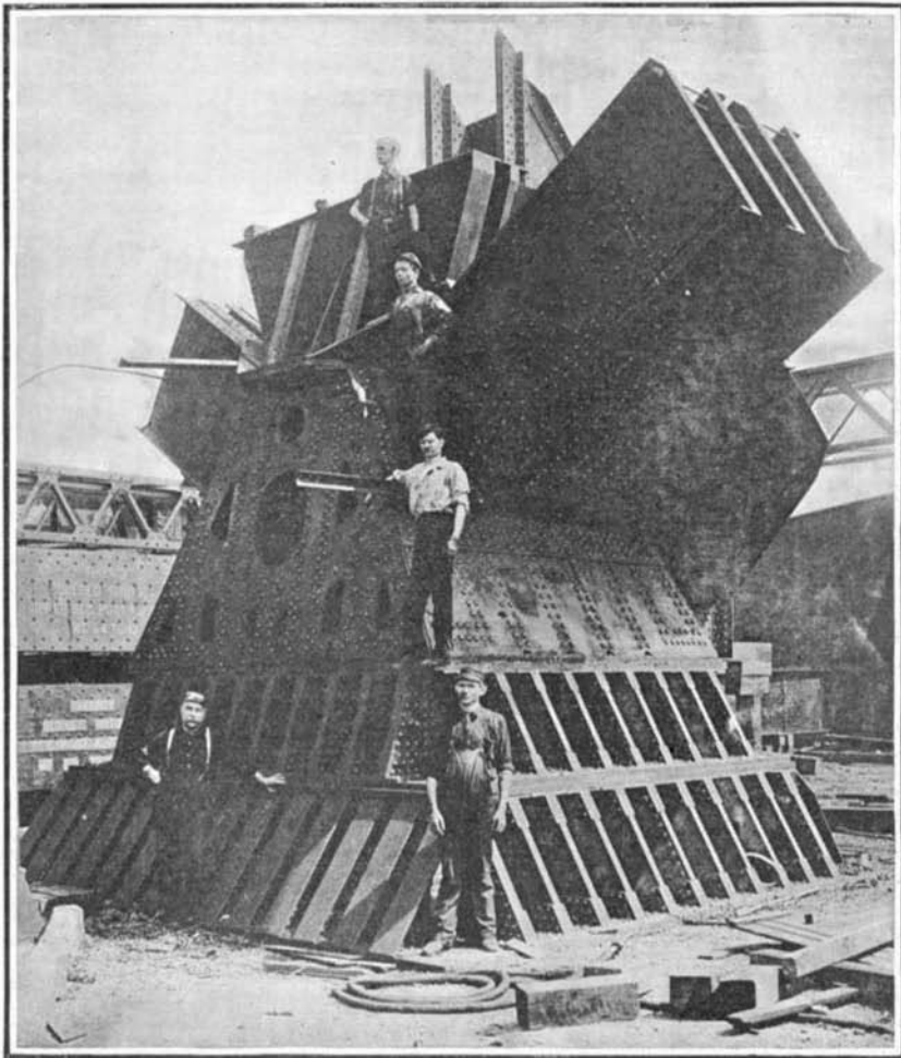
One of the Four Pedestals and Main Shoes Which Carry the Whole Weight of the Bridge. Weight 278 Tons.
