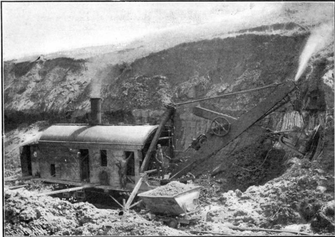
Digging Out Shale With the Steam Shovel.
