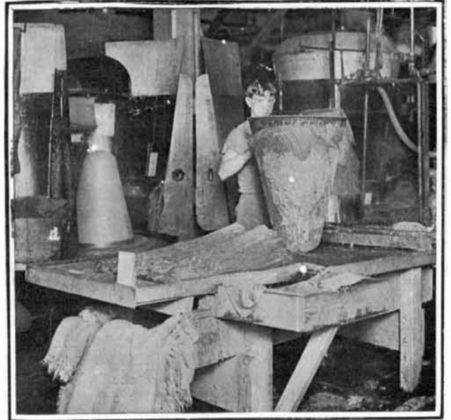
Stripping Body from the Cone After Forming.
