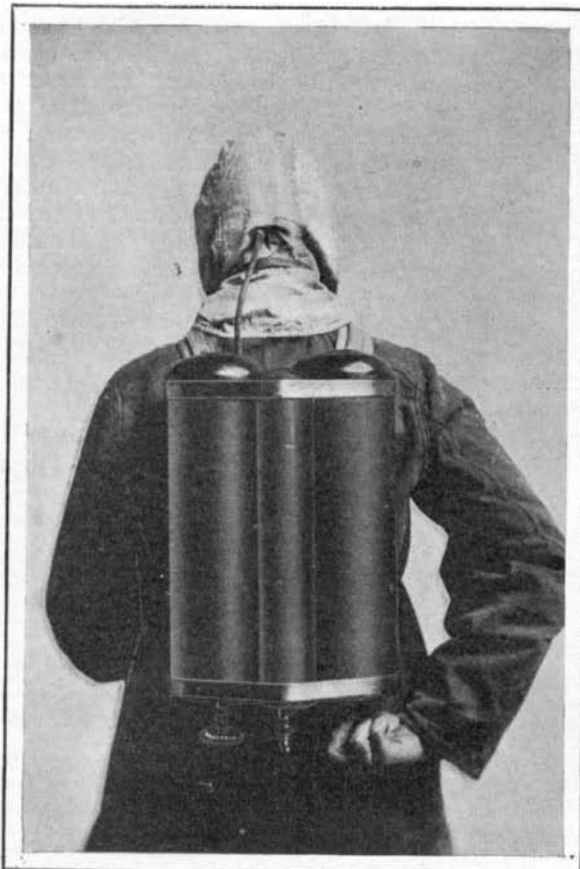
An Air Cylinder is Strapped on the Back of the Fireman. Enough Air is Carried to Last an Hour.
