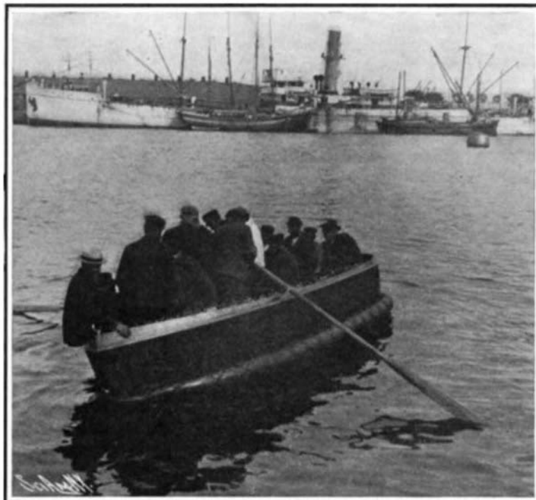
TWENTY-ONE-FOOT COLLAPSIBLE LIFEBOAT EXPANDED. Twenty-two men are trying to list her over.
