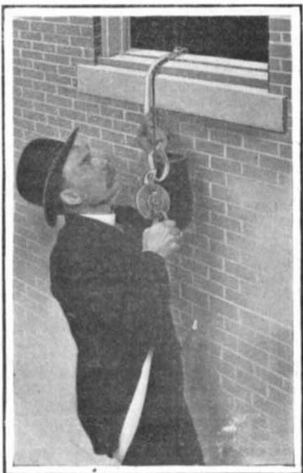
METHOD OF USING THE FIRE ESCAPE.
