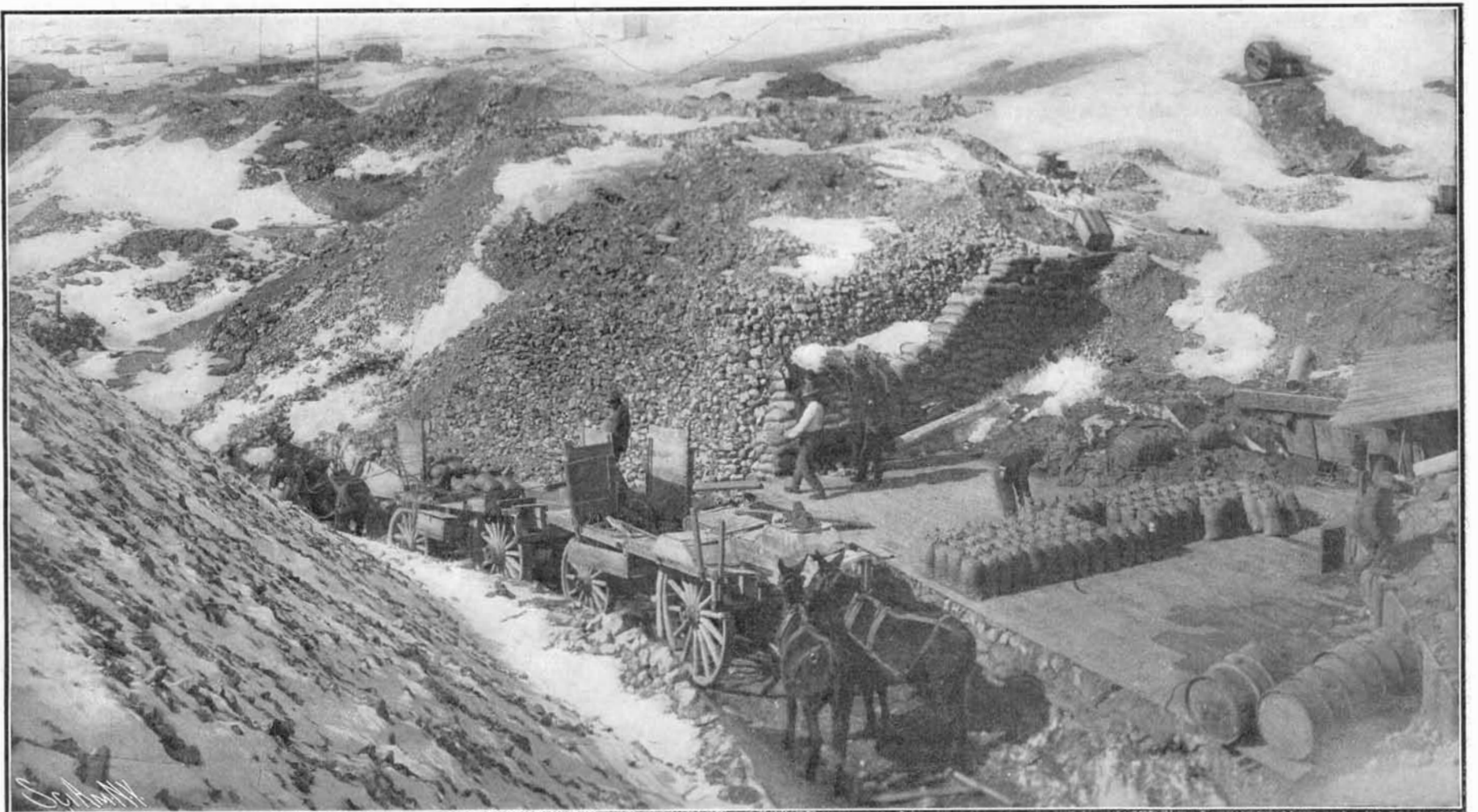
Loading Sacks of Gold and Silver Ore on Wagons for Shipment to the Smelters.
