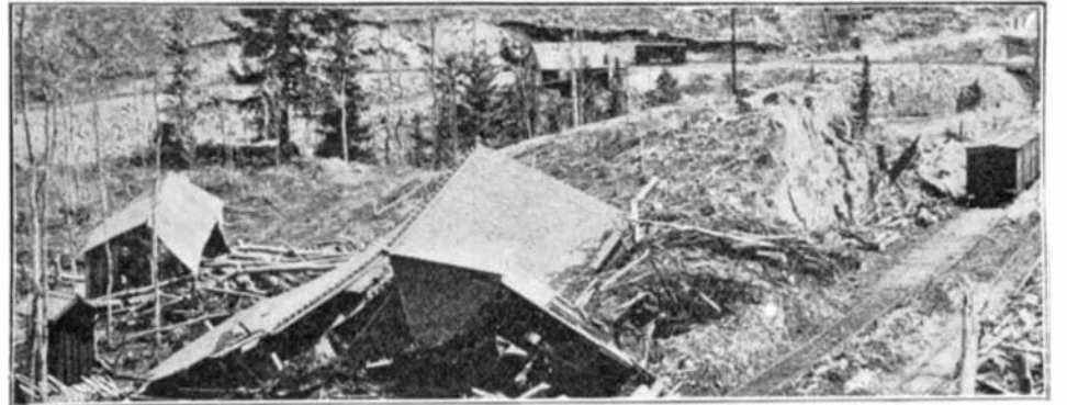
Ruin Caused by an Avalanche at Amer, Colorado.
